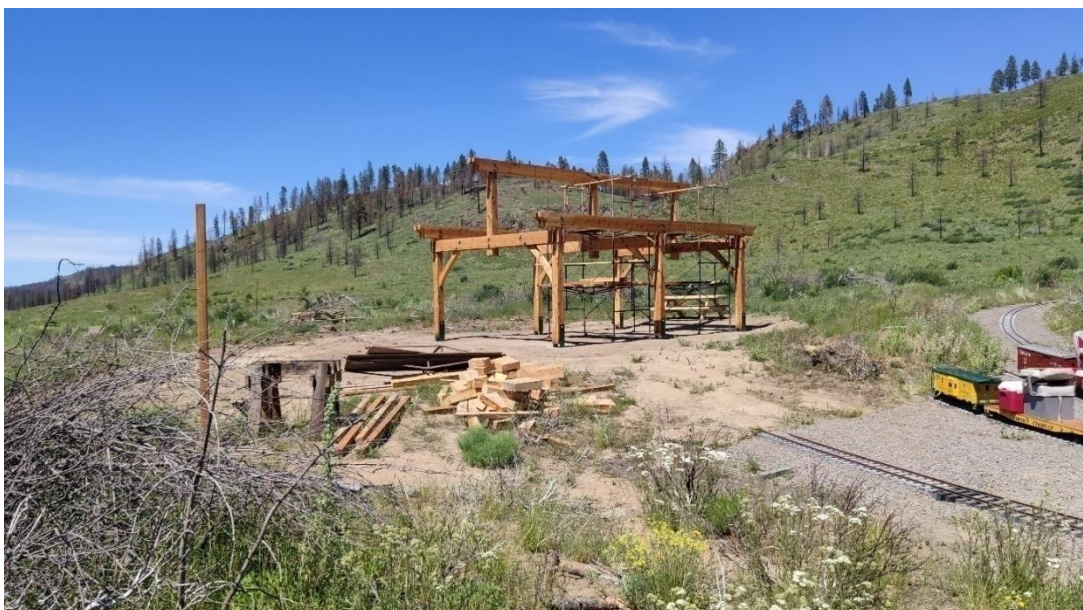
As there is now no shade, a pergola is being built.
